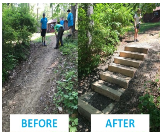
Infiltration steps installed by 30MRWA's YCC allow stormwater to soak in, filtering it and reducing erosion.
