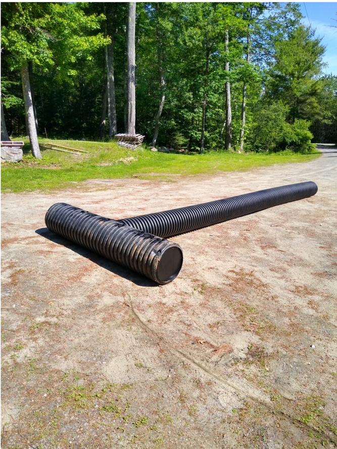
The beaver deceiver is a 20-foot by 12-inch black PVC culvert with a 6-foot by 15-inch piece of culvert attached to it to form a tee. The ends of the tee are blocked
